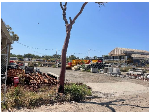
Figure 11: Overview of Miller Road access point showing industrial waste, buildings, concrete and gravel road base. Note levelled ground surface.
